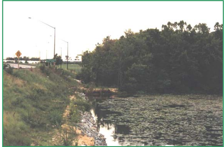
Storm water management pond serving the US 301 MD 5 intersection at the northern edge of the Sub-Area.
