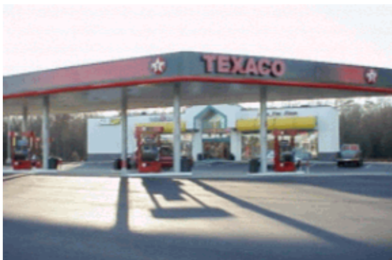
New Gas/Convenience Center Located at Intersection of MD Route 227 and US 301
